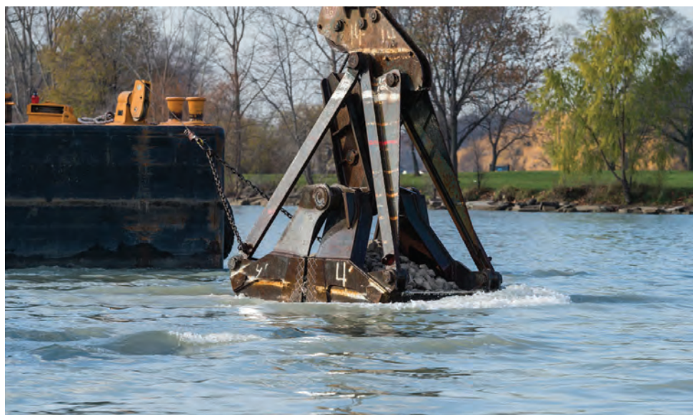
Loaded buckets were lowered to the river bottom before the rock was released. The latest Belle Isle reefs are located in water that is 18 to 22 feet deep, and they rise about 2 feet above the river bottom. About 4 acres of new rock reefs were created and are located outside commercial shipping channels. Image credit: Austin Thomason, Michigan Photography
